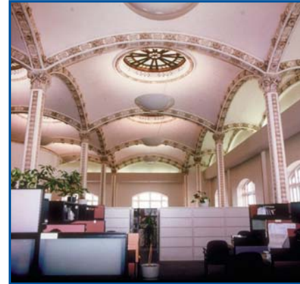
SonaSpray "fc" furnishes this office with a pleasing ceiling finish.
