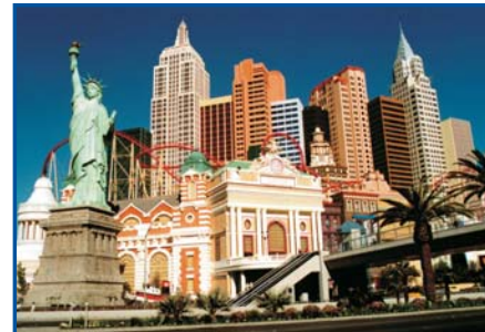
Celbar helps to control sound transmission between the walls of this Las Vegas hotel.
